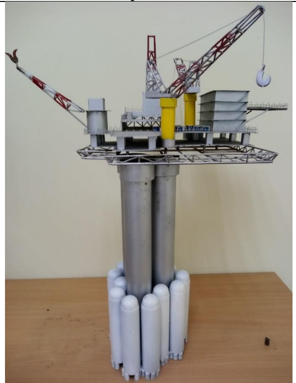
CONCRETE GRAVITY STRUCTURE Water depth: 50-400m
